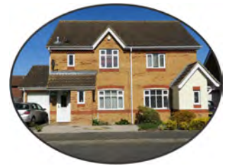
Different finishes help distinguish each house in the pair
