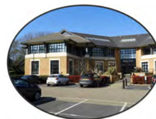
Offices at Parsons Green
