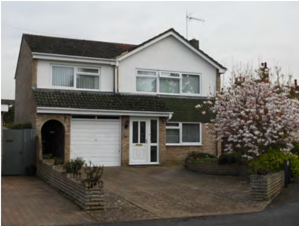
Green hanging tiles and partial rendering provide soft finishes with the detached house set back sufficiently to allow on plot parking
