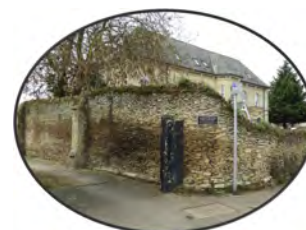
Priory barn walls
