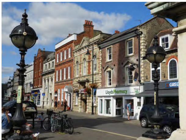
Market Hill has a strong historic character with many individually designed and now listed buildings
