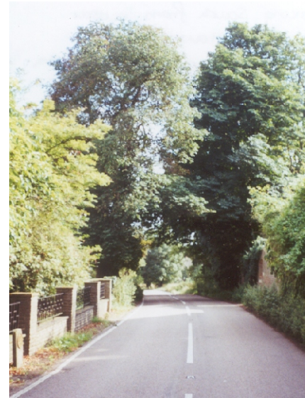
A long view looking South along Raunds Road
