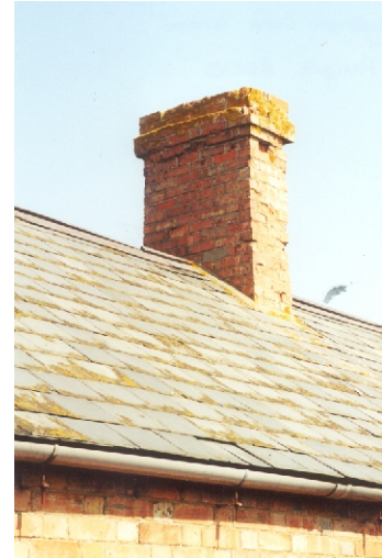
An unelaborate chimney detail typical of those found in Keyston
