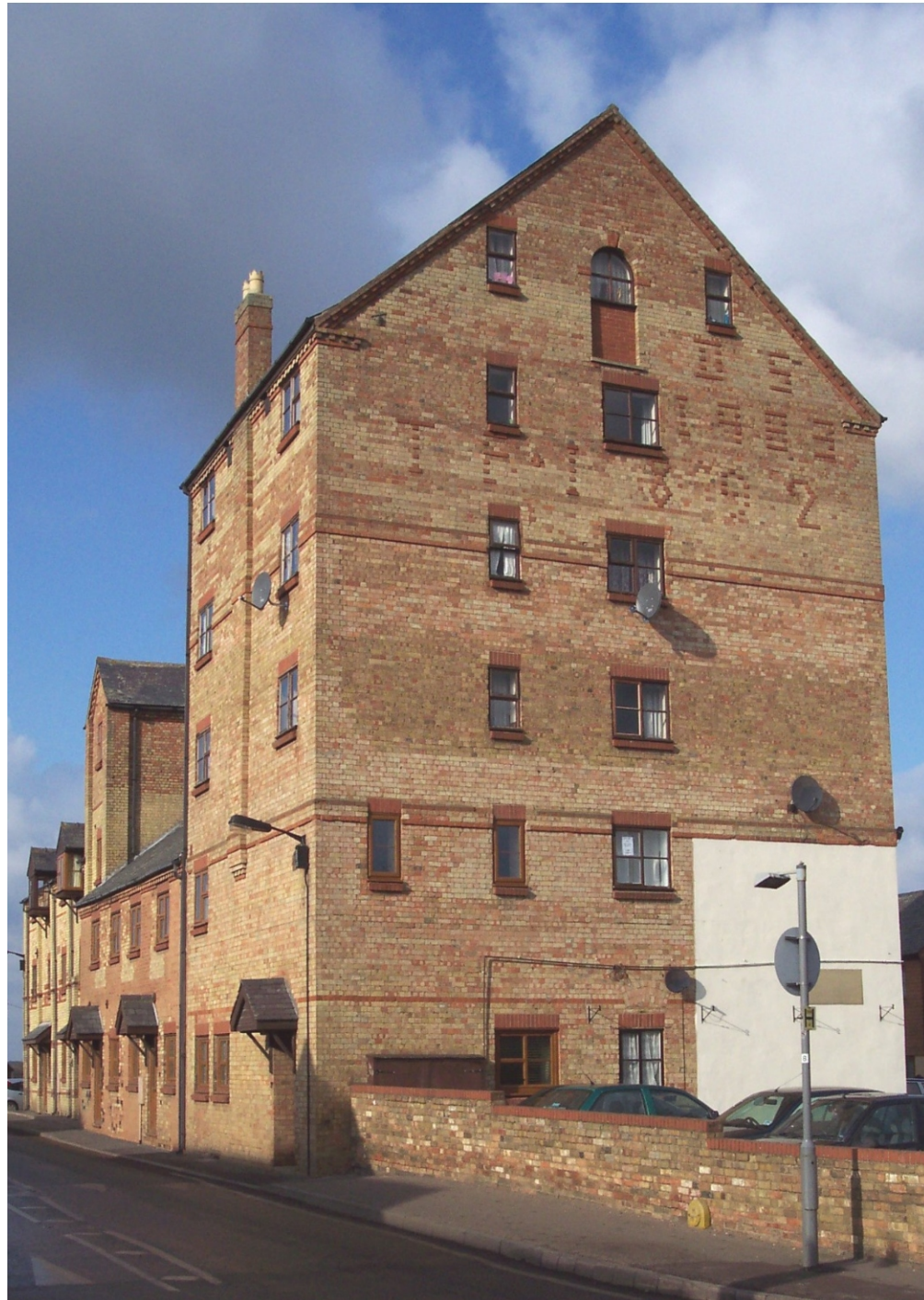
Mill. The six storey building forms a landmark at the north end of Great Whyte. It has simple gables forms and the openings are regularly spaced on the elevations. Window details are simple.
