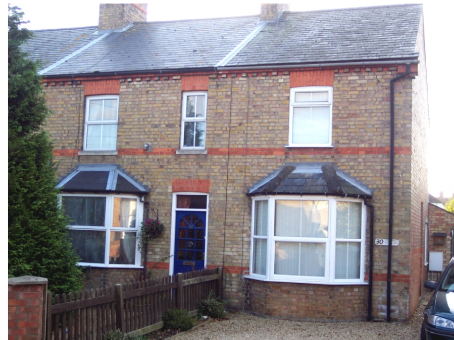
Blenheim Road. A slightly 'grander' terrace, with front bay, red-brick detailing and dentilled eaves.
