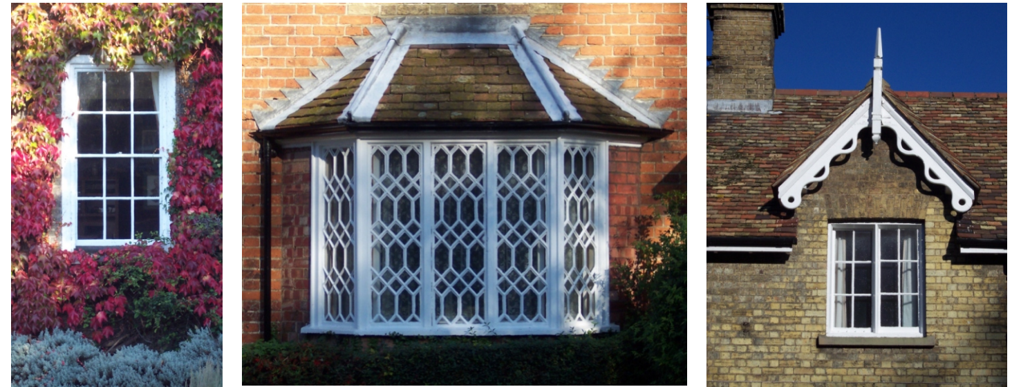
Church Green. The neo-classical 12 pane sash is mixed with ornate bargeboards of Gothick origins. The two styles, and the range of materials and scales, bring great variety and visual interest to this part of the Conservation Area. External materials include stone, in Abbey Green, to gault and soft red brick. Roof materials are the local clay peg tile mix and natural slate.
