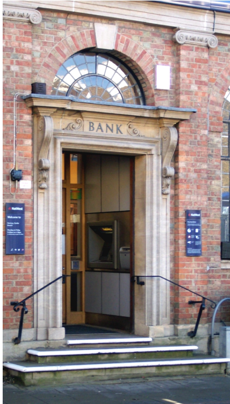
High Street. An elegant neo-classical doorcase and fanlight in a former dwelling, and a more ornate version on a commercial premises.
