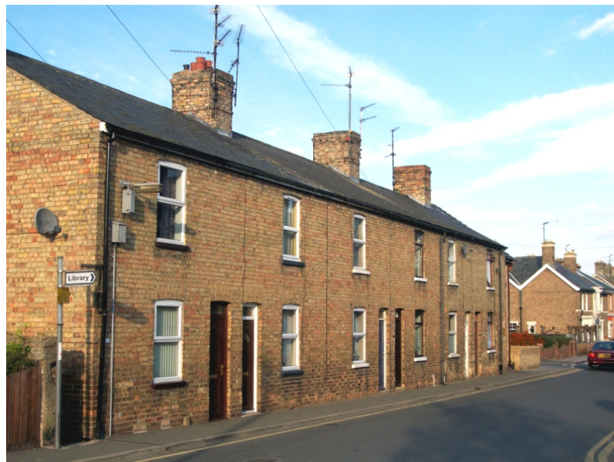
Whytefield Road. Modest terraces in gault brick and slate. Unfortunately, all the original window and door detailing has now been replaced.
