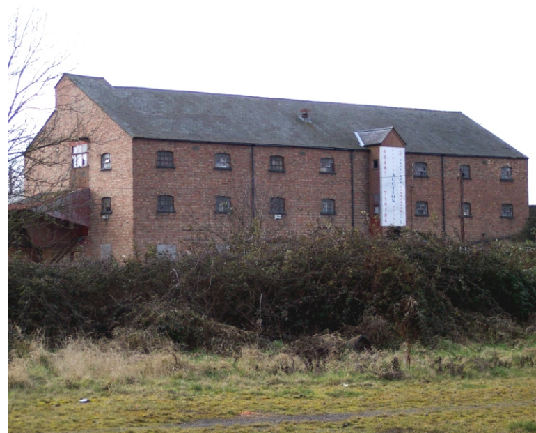
Railway warehouse. Large scale, regular openings and brick and slate brought to the town on the railway.
