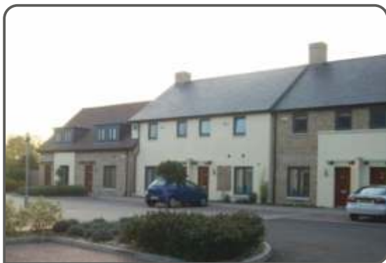
Small scale brownfield redevelopment showing good use of materials and scale (Thrapston Road, Brampton)
