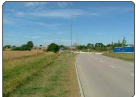
4. View along Cambridge Road from the east
