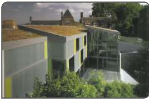
Green roof system to help deal with intercepting rain water
