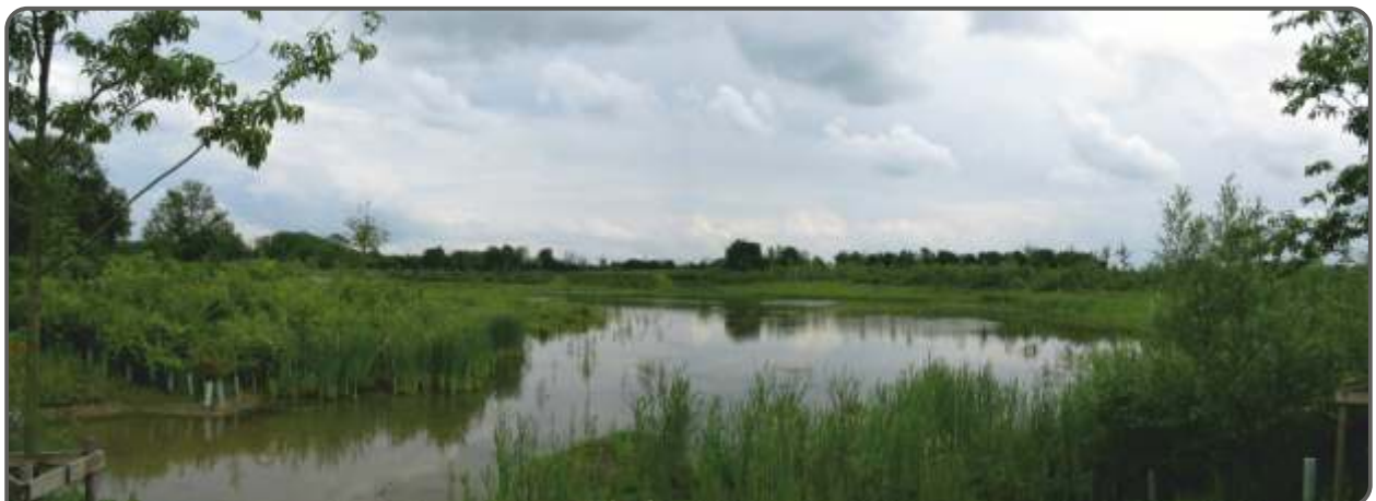
Existing flood attenuation pond at Love's Farm
