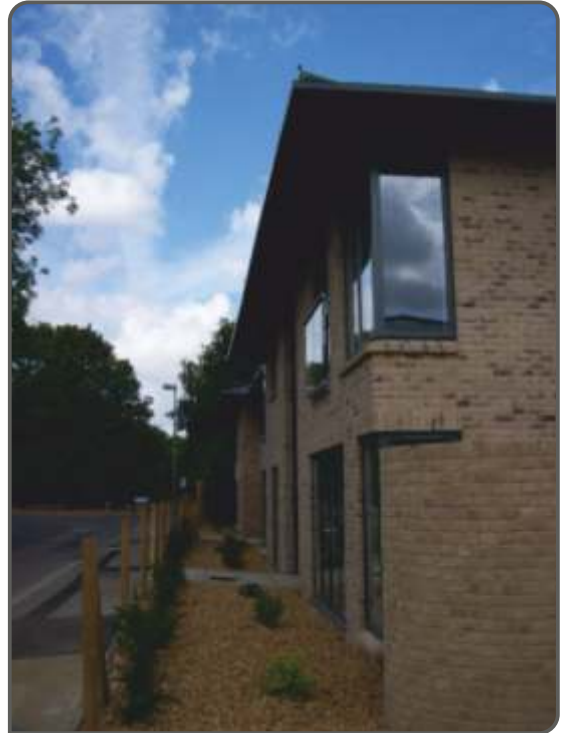
Architectural detailing (Station Road, Ramsey)
