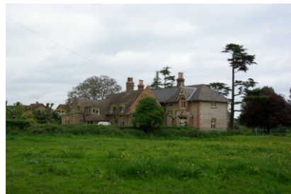
16th & 17th Century manor house, Bury
