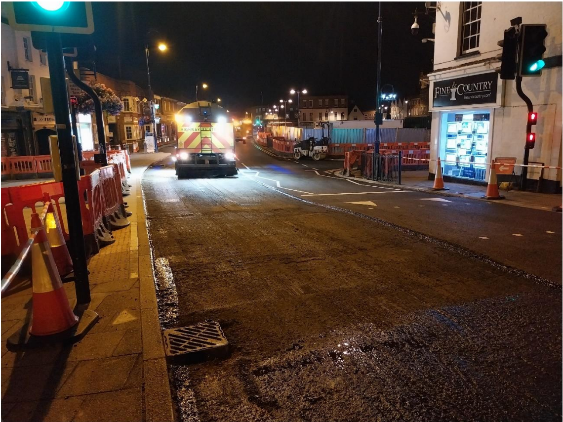
14/08/2024 – Carriageway resurfacing works continuing on High Street and bridge
