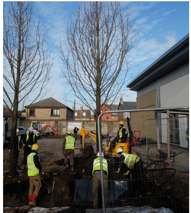
Mature lime trees retained at Rowley Arts Centre, St Neots
