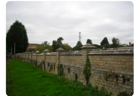
(F). Wall of former formal gardens. This wall acts as a retaining wall to land to the north on the other side
