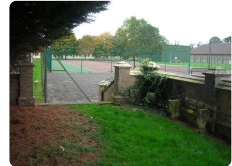
(F). Wall with steps. Former integral seat along wall edge is missing
