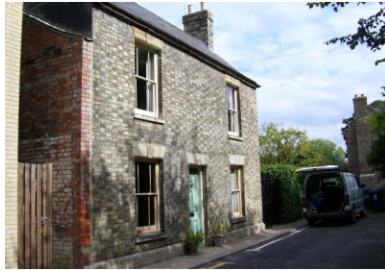
A. Wood Street
