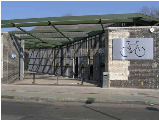
Finsbury Park Cycle Station – access is made secure by the use of smart card control
