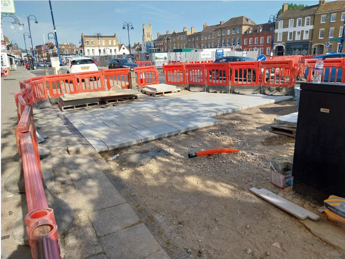
30/07/24 – Repaving outside Nationwide in York Stone
